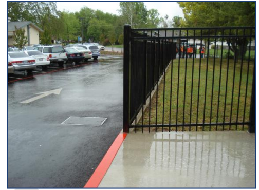
Figure 7 The newly constructed sidewalk does not reach the road. Walk audit participants, seen through the fence in orange, are standing at the end of the school driveway on Corta Way.
